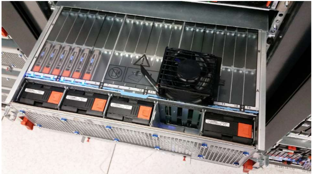
Figure 21. Fan in the 120-drive DAE
