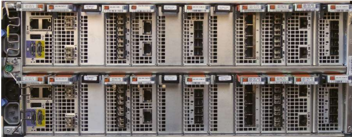
Figure 33. Back view of the SPE with SPA (on the bottom) and SPB (on the top)
